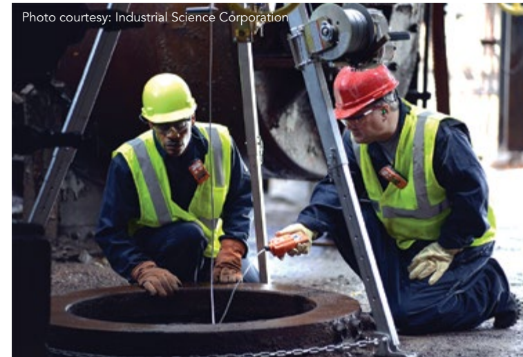
Photo courtesy: Industrial Science Corporation A "permit-required confined space," as defined by OSHA, may have no hazardous atmosphere within the space whenever any employee is inside. This is the impetus for using a multi-gas monitor to perform atmospheric testing, prior to entering a confined space.
